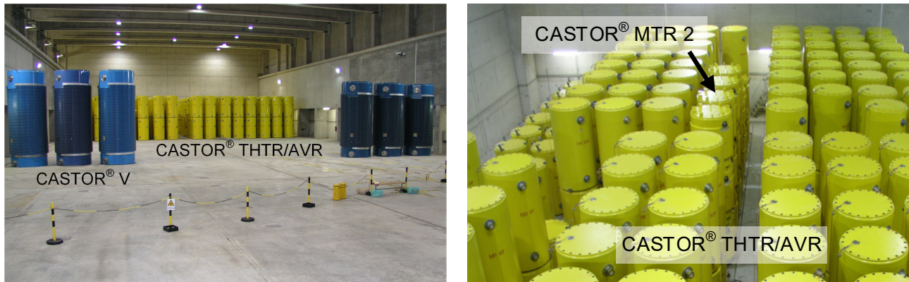
Figure D-5: View into the Ahaus spent fuel storage facility (Copyright: BGZ)
