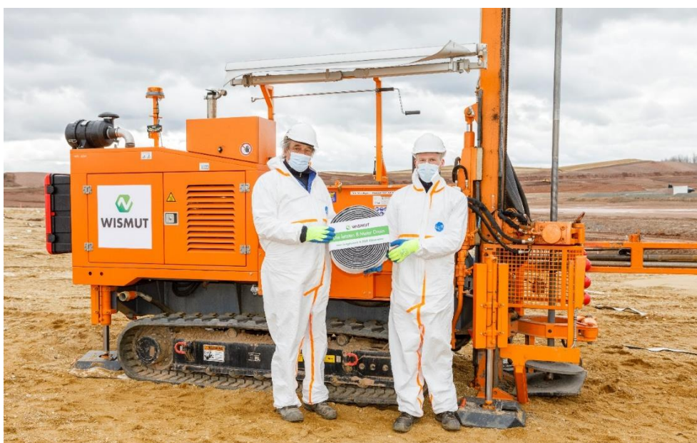
Fig. 1: The last drainage wick was installed in Basin A of the Culmitzsch industrial tailings pond in 2021 (Copyright: Wismut GmbH)
