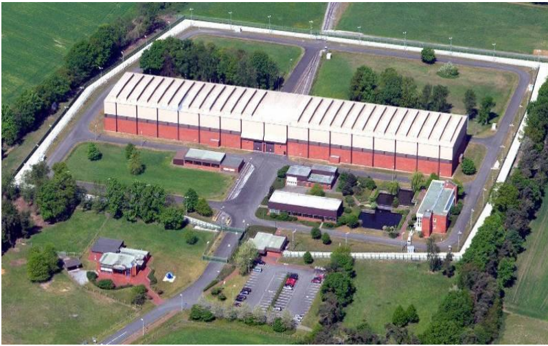
Figure G-1: Ahaus storage facility (Copyright: BGZ)
