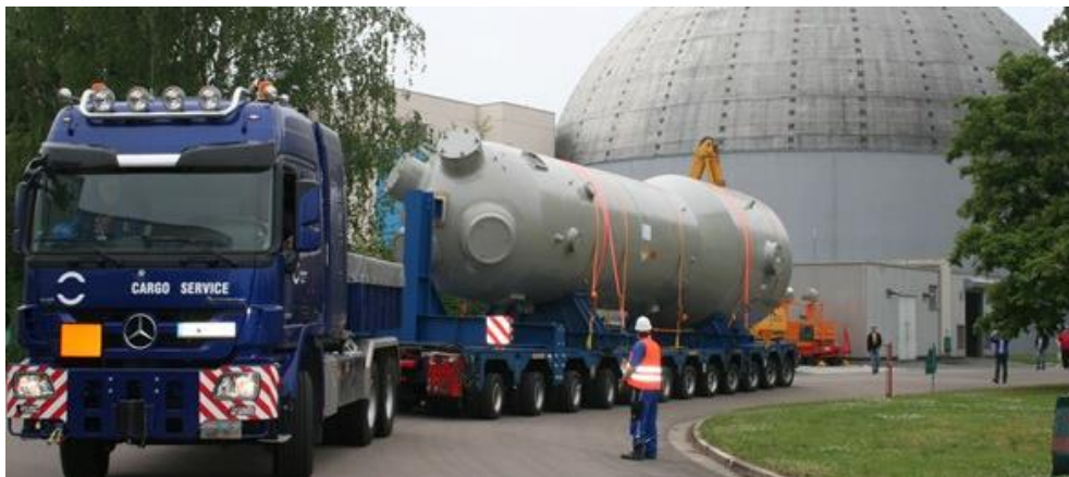
Figure D-20: Removal of the steam generator from the Obrigheim nuclear power plant (Copyright: EnBW)
