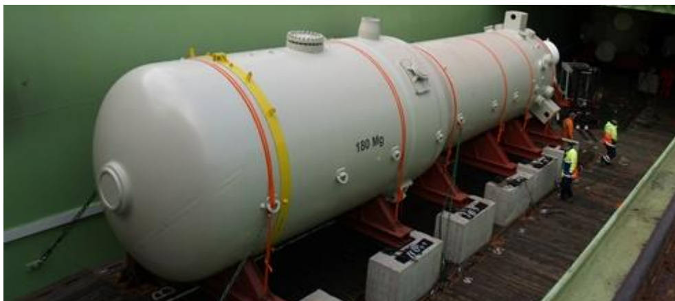
Figure D-20: Removal of the steam generator from the Obrigheim nuclear power plant (Copyright: EnBW)
