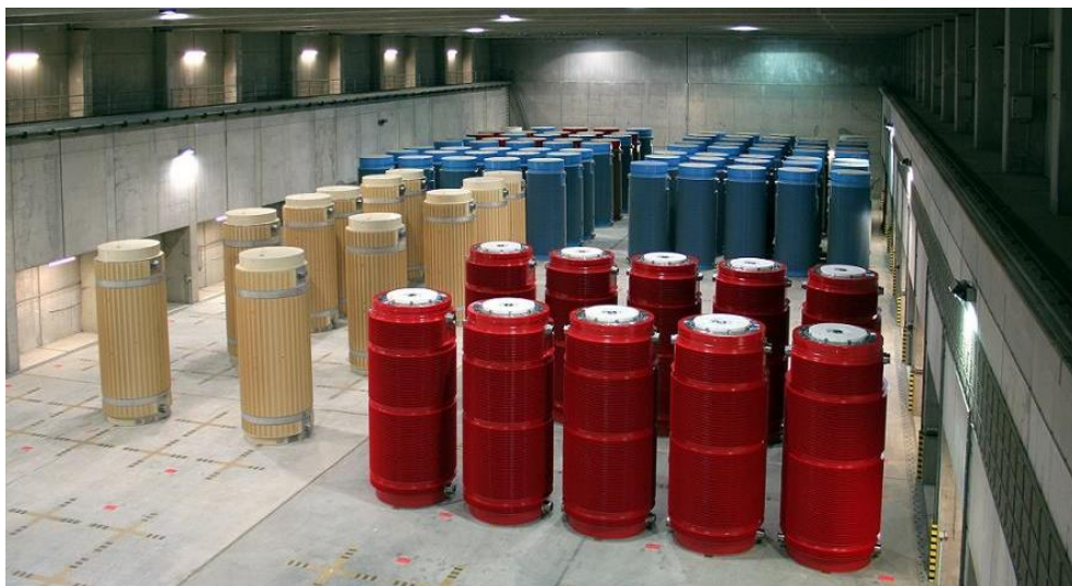
Figure D-3: View into the Gorleben spent fuel storage facility (Copyright: BGZ) Transport and storage casks of various types
