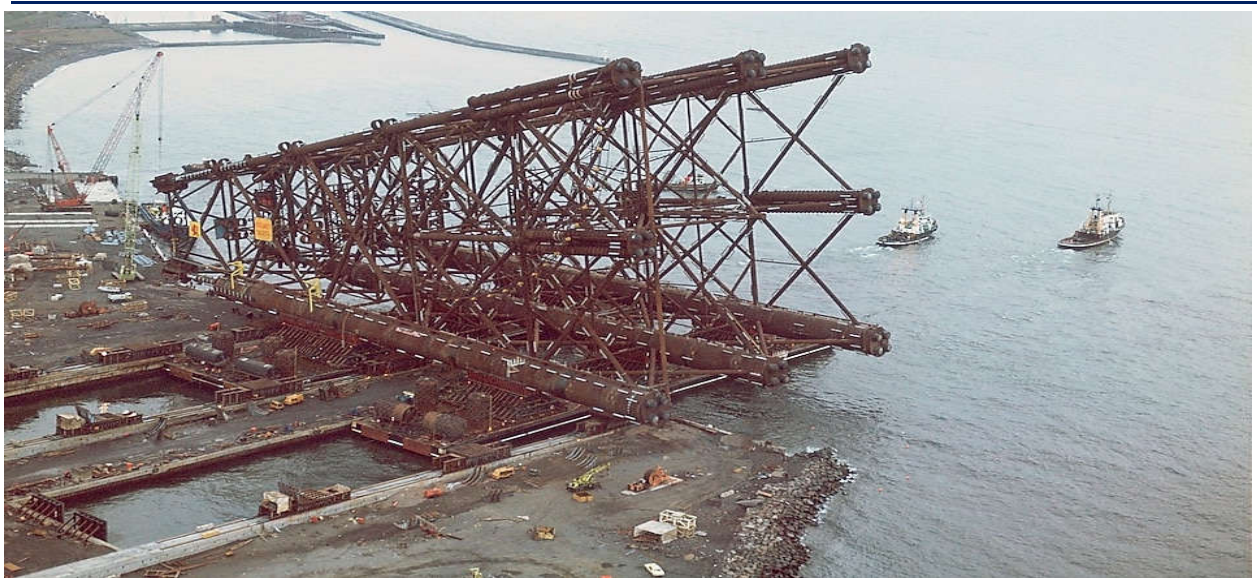
Figure 7 Brent Alpha Jacket at Load Out for Installation (from Shell Brent Alpha Jacket TD - BDE-A-JKT-BA-5801-00001)
