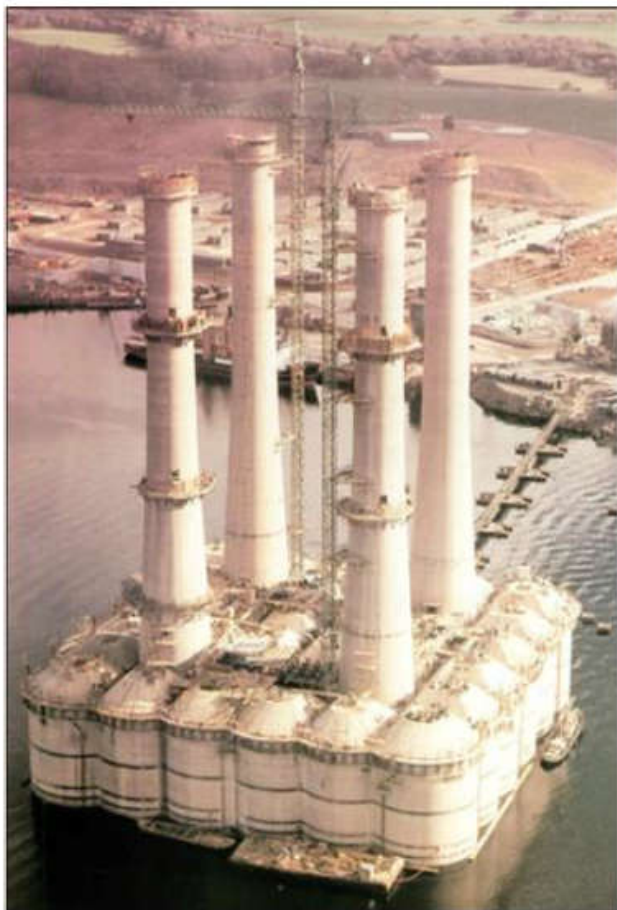
Figure 7 Brent Alpha Jacket at Load Out for Installation (from Shell Brent Alpha Jacket TD - BDE-A-JKT-BA-5801-00001)
