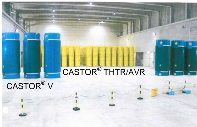
Figure D-5: Ahaus transport cask storage facility (TBL-A) (Copyright: GNS) left: CASTOR® V and CASTOR® THTR/AVR right: CASTOR® MTR 2 between CASTOR® THTR/AVR
