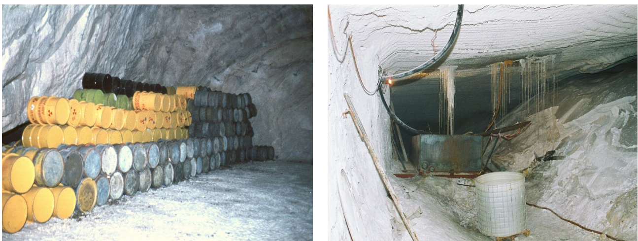
Figure D-13: Asse II mine (left: waste package in an emplacement chamber (no more accessible today), right: dripping point) (Copyright: BfS)
