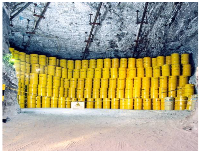
Figure D-10: Repository for radioactive waste (ERAM) (left: aerial photograph, right: emplacement chamber with stacked low-level waste drums) (Copyright: BfS)
