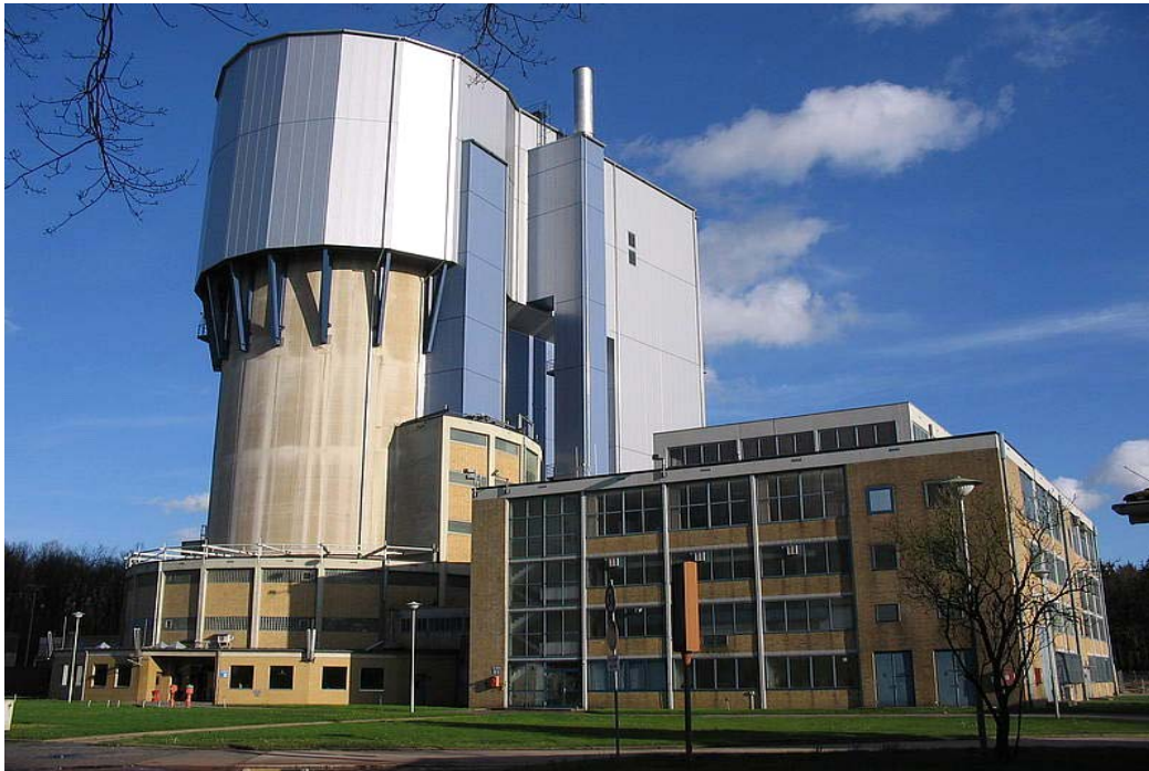
Figure D-17: AVR reactor building with material lock (Copyright: EWN)
